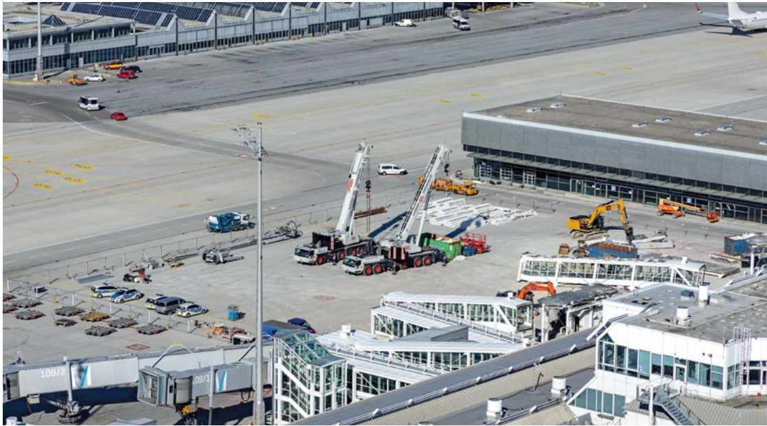
Construction works started on the western apron in early March 2019.
