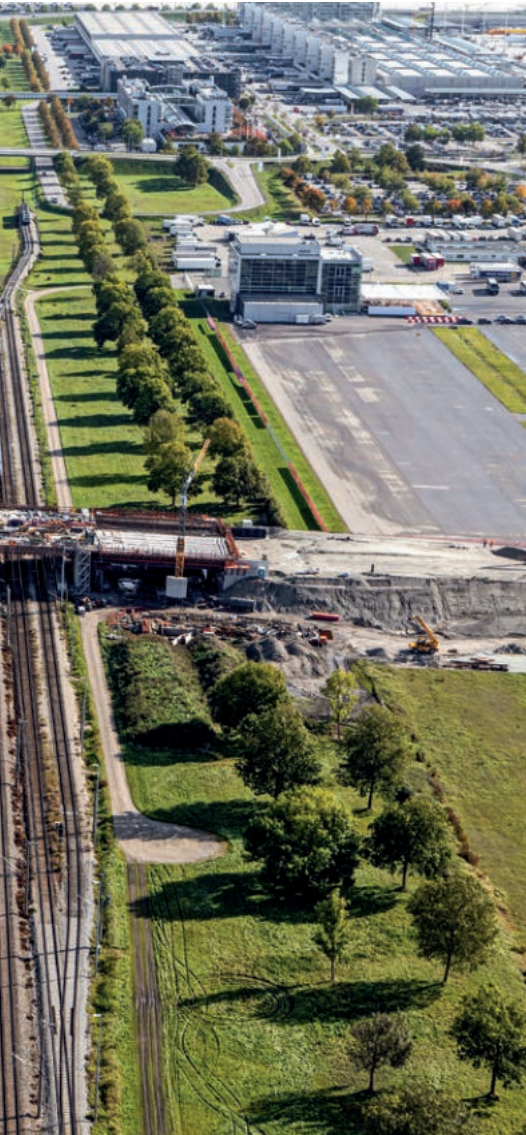
A new bridge is being constructed to the LabCampus over Zentralallee.
